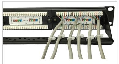
Secure the cables tightly on the support bar
